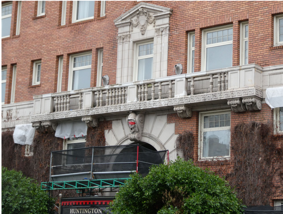
Photo 21. Work In Progress. North elevation detail showing select third floor balcony balusters removed for repair and reinstallation and/or replacement
