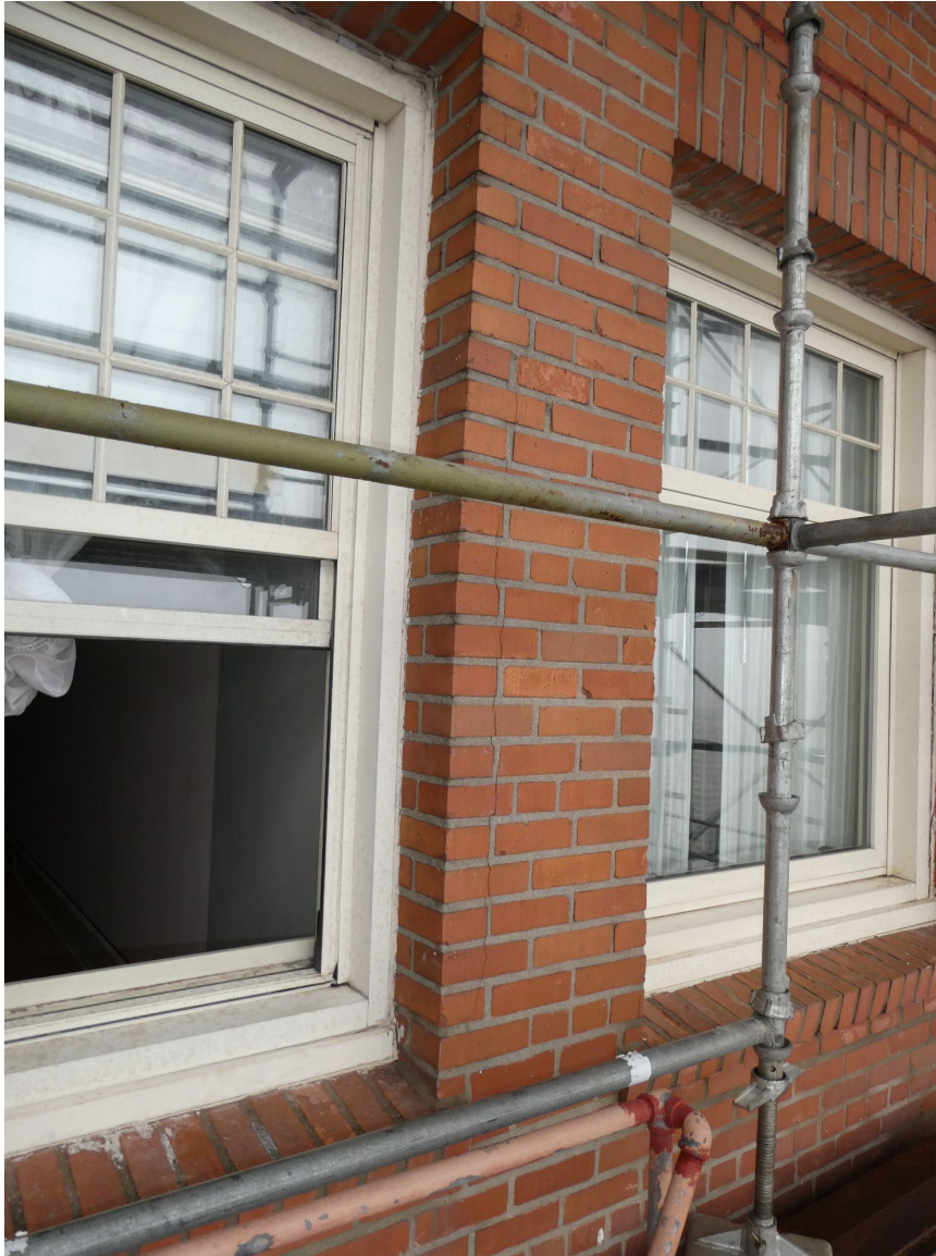
Photo 23. Work In Progress. Detail of brick repair at Twelfth floor
