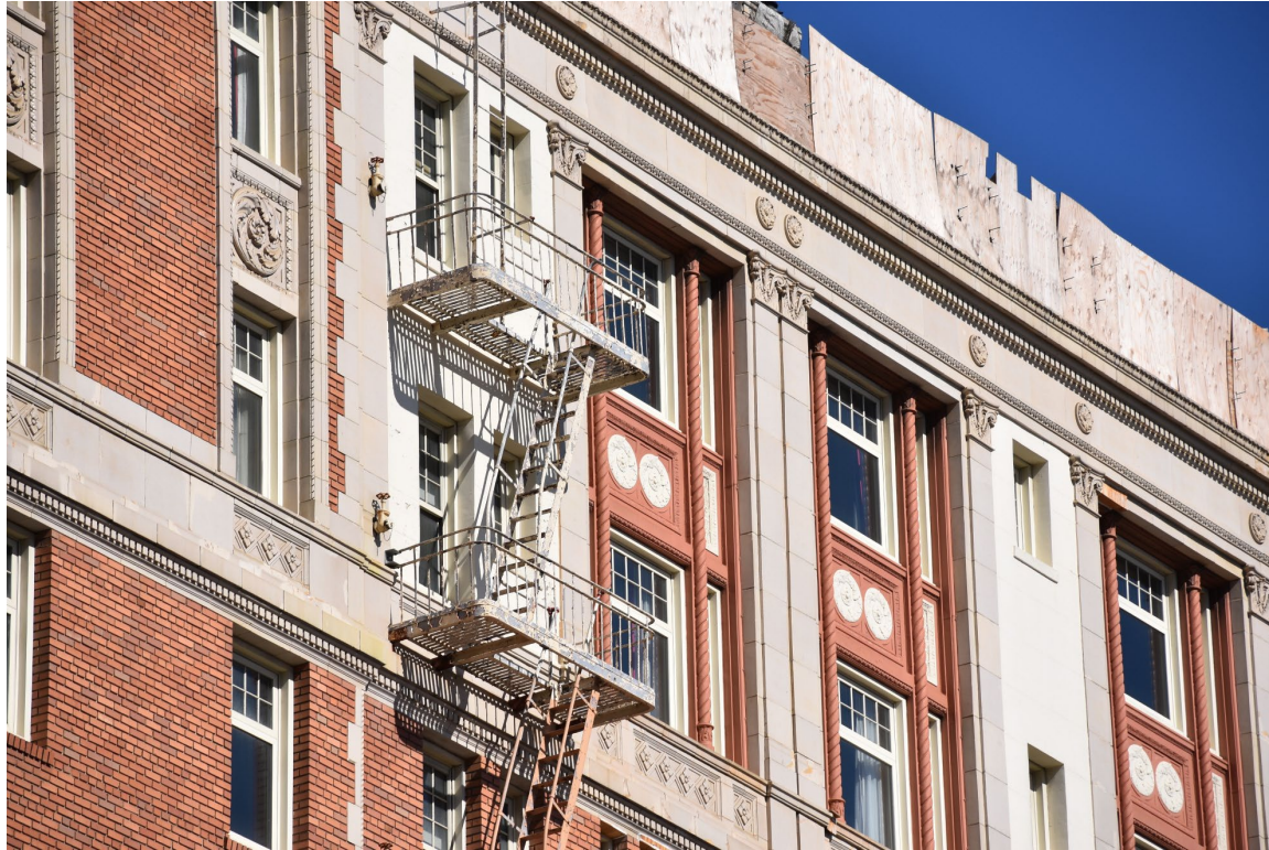
Photo 6. West elevation, detail at 11th and 12th floors showing decorative pilasters and friezes between (replacement) windows
