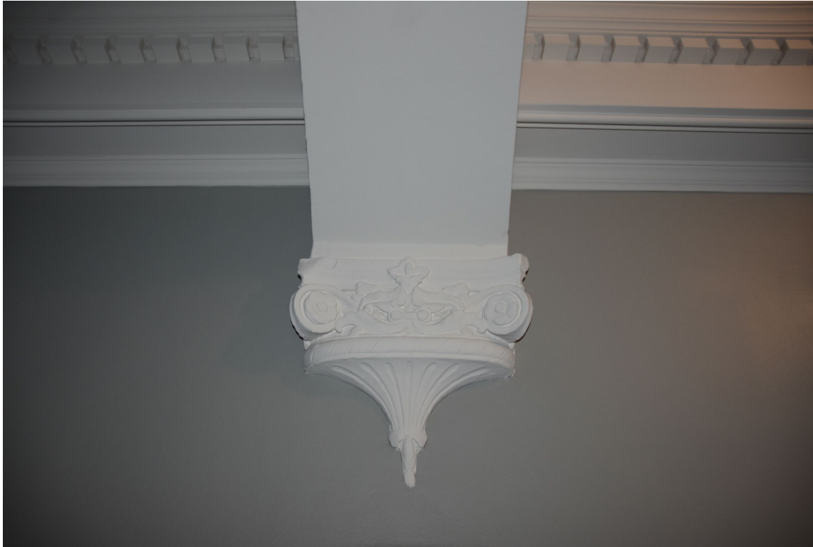
Photo 18. Detail of arched beam with original ornamental floral plaster cap. Typical of upper floor corridors
