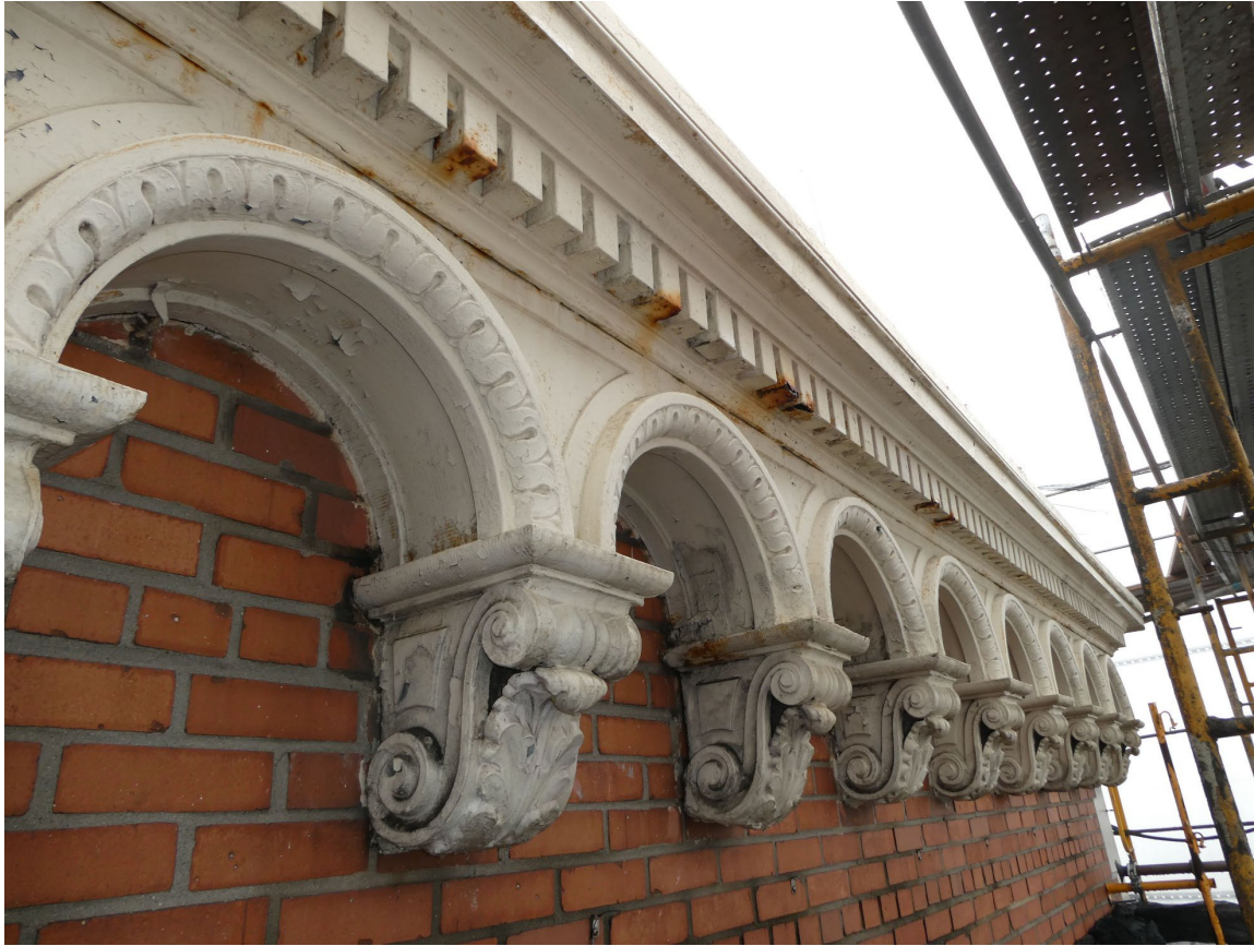
Photo 22. Work In Progress. Detail of brick and terra cotta repair at Twelfth floor
